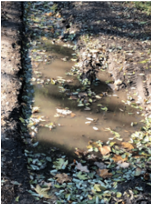
Figure 6: Ruts caused by cars parking on the verge of the Centennial Garden
